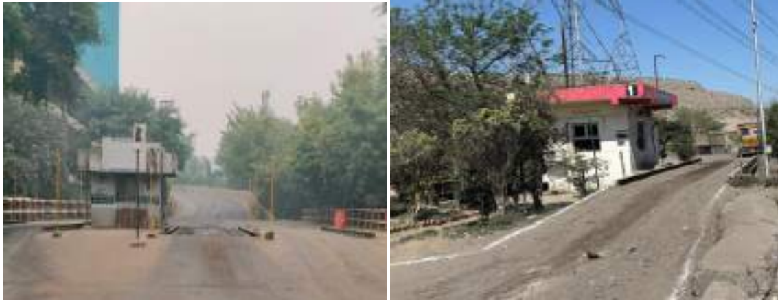
Figure 3: Weigh Bridge Section of a WtE Plant
