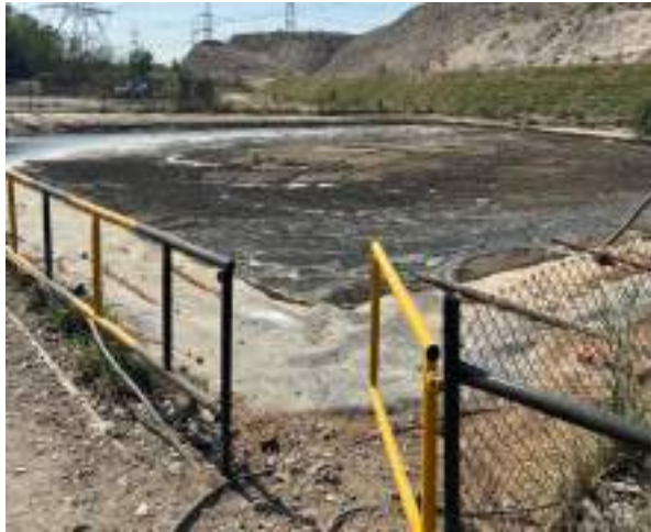
Figure 17: Leachate Collection Pond
